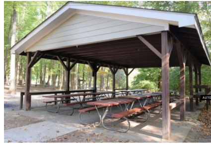
Nottoway Park, Shelter A
