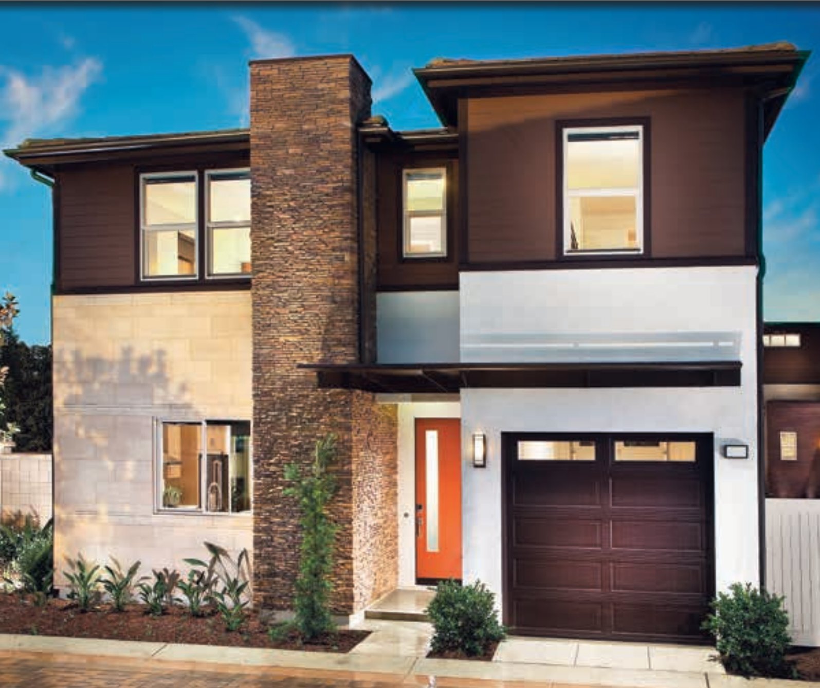
(Left Wall) French Limestone with 6" Chiseled Limestone Band - Country Beige (Center Column) Mountain Strip Stone - Chablis
