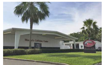
Martin's Collision Center is well-known for high-quality work, which is why it chose USI America for its spray booths.
