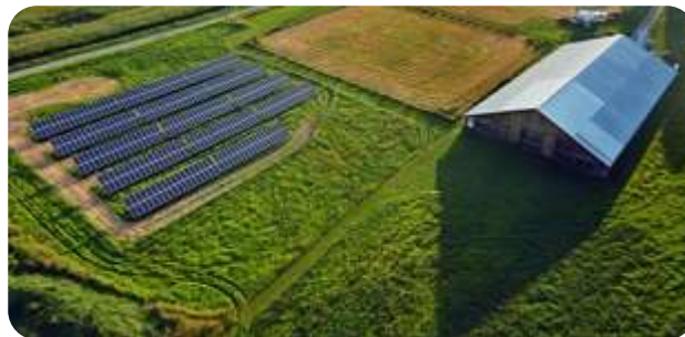
Agriculture: water pumps, remote processing plants and facilities
