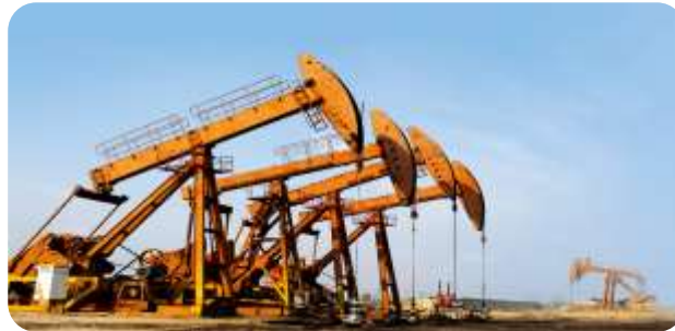
Oil & Gas: oil, gas and water wells RTU, TETRA, CP, Decarbonization
