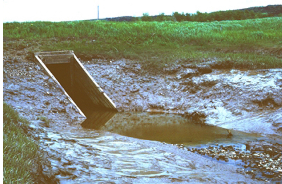
Aboiteau—sluice gate
