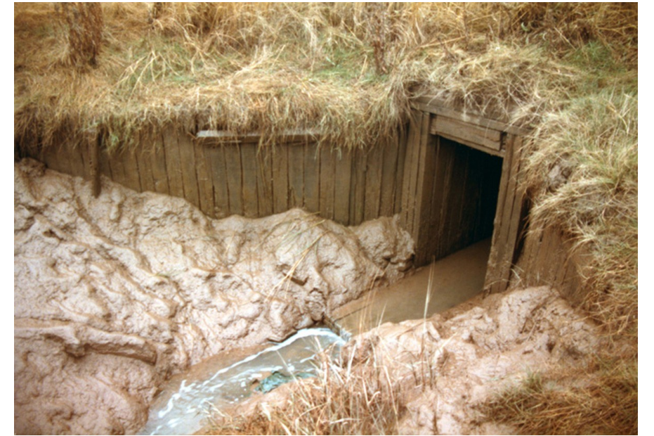
Aboiteau—sluice gate
