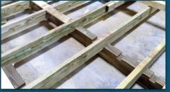
12" On-Center Floor Joists 16" OC is Standard
