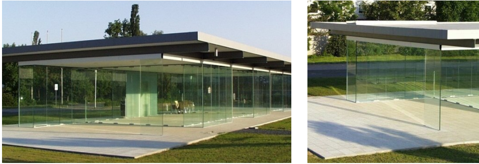
Figure 4-1 Centre of German Glazing handcrafters in Rheinbach, Germany
