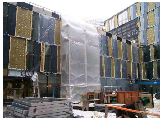
Figure 34: Temporary exterior heating via test specimen.
