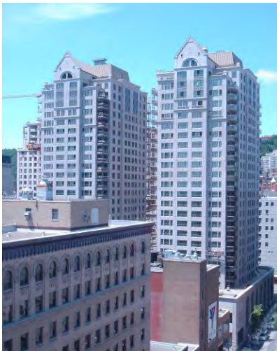
Figure 3: Aluminum punch windows and precast concrete (Montreal, QC)
