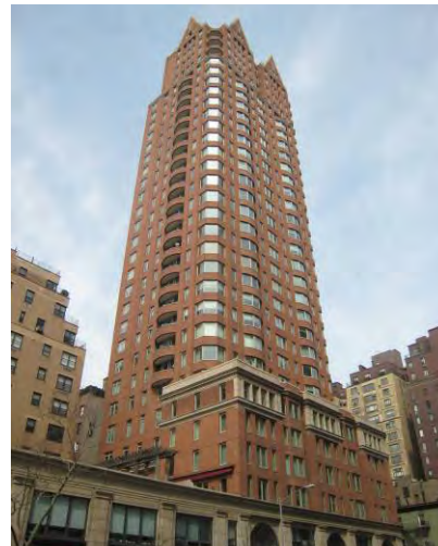
Figure 4: Aluminum punch windows and brick cladding (New York, NY)
