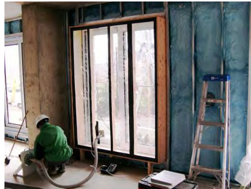
Figure 21: Interior test chamber used to test a punch window assembly
