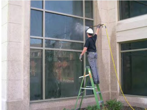
Figure 35: Diagnostic hose testing of curtain wall section.
