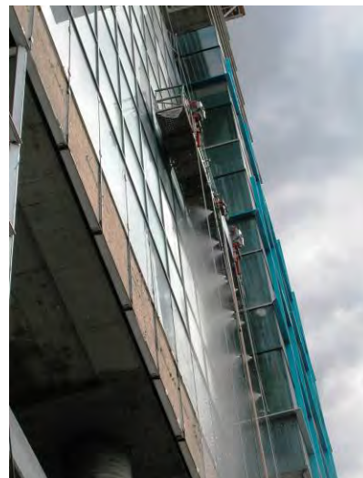
Figure 13: Field testing for resistance to water penetration.
