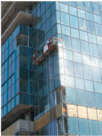
Figure 31: Calibrated sprinkler rack hung from suspended scaffolding.
