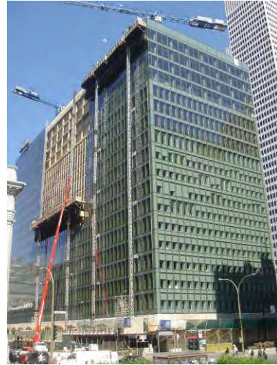
Figure 2: Metal & glass curtain wall - building reclad (Montreal, QC)
