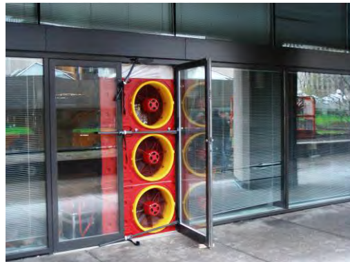
Figure 23: High power blower door installed within a confined space adjacent to an exterior wall.
