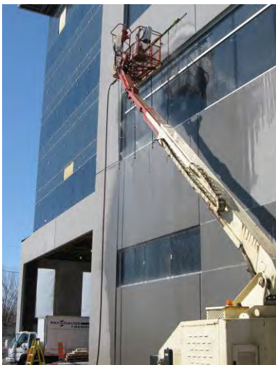
Figure 12: Field testing for resistance to water penetration.
