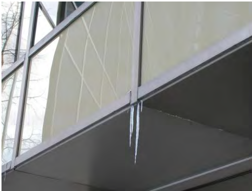
Figure 7: Example of exterior icicle formation due to excessive air exfiltration within a curtain wall assembly.
