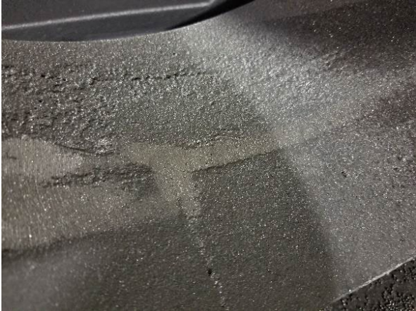
Interior casting surface, close-up
