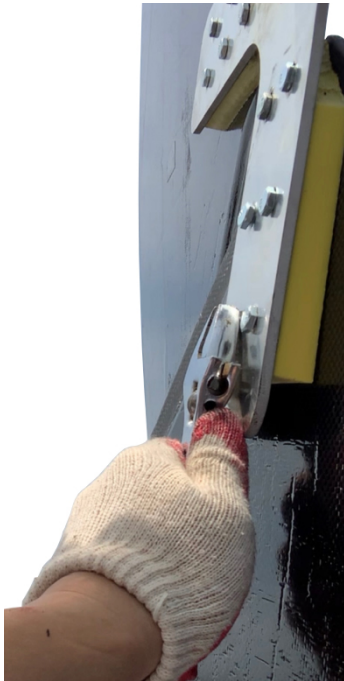
Figure 2.9: Ensure the nuts are tight with plastic washers against the carbon.
