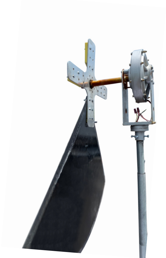
Figure 2.10: Mount blades 2 persons one at a time with brake on
