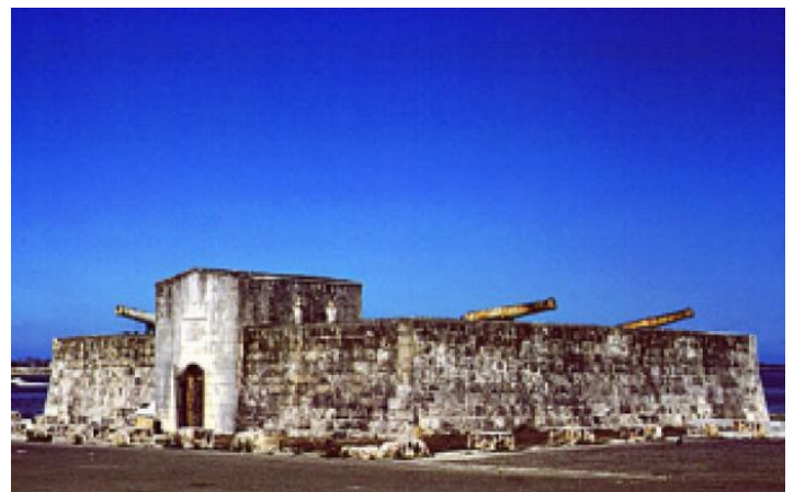
Originally built in 1742, Fort Montague still stands east of Nassau
