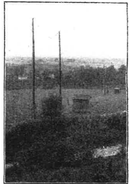
The sending and receiving huts of the very short-wave station of the Post Office at Weston-super-Mare. Communication is maintained across the Bristol Channel.
