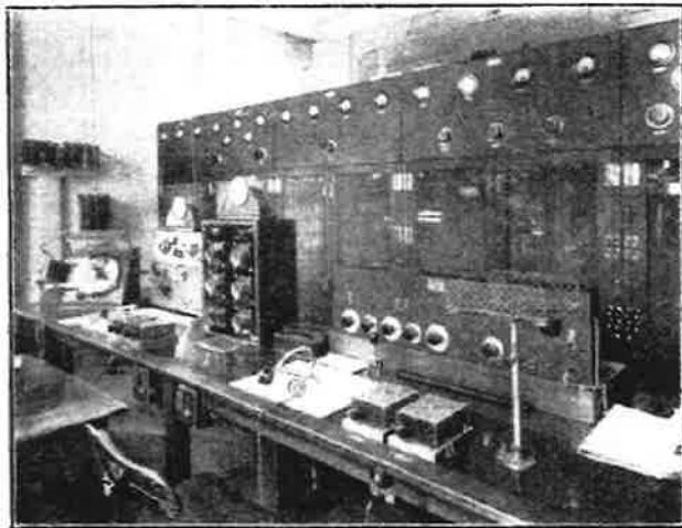
The operating bench at Land's End station with the transmitter in the background.
