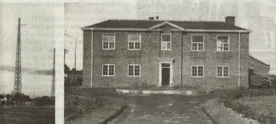
Highbridge receiving station, original entrance and main building
