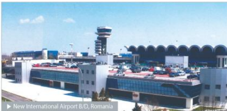
► New International Airport B/D, Romania
