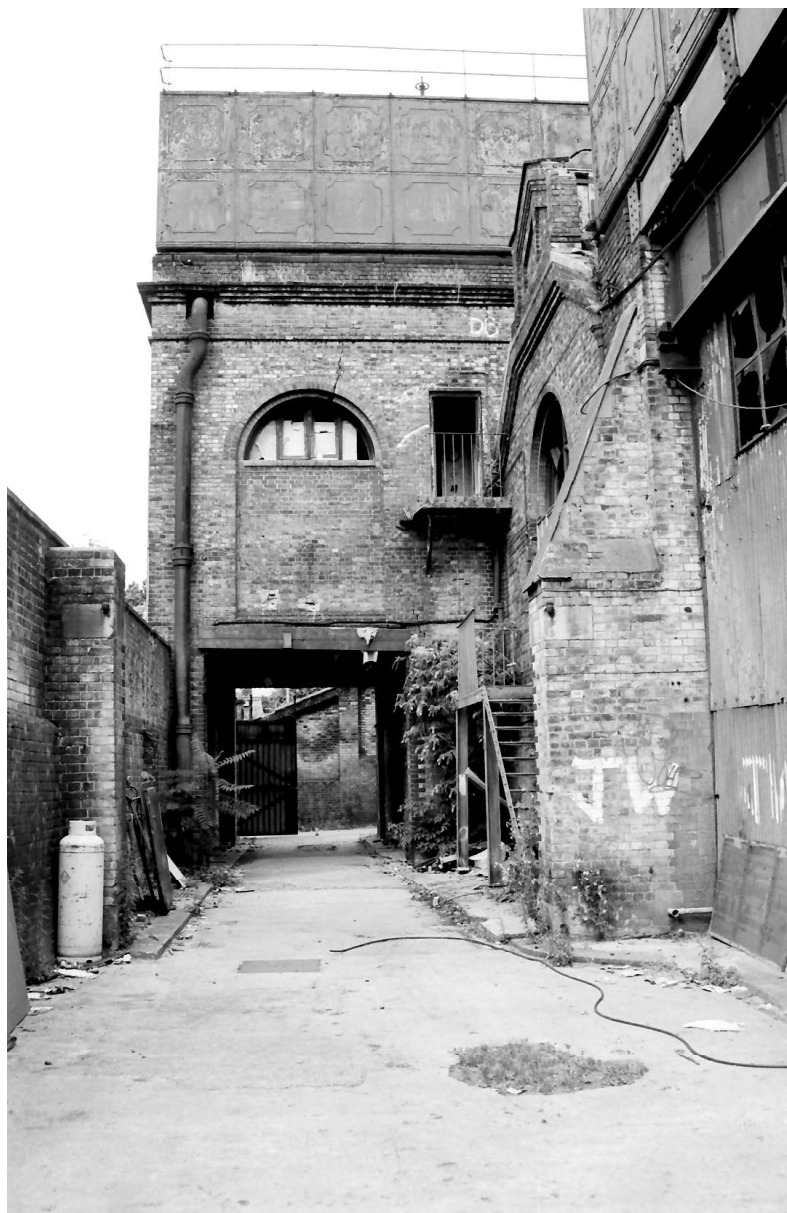
Figure 3. The yard to the north of the boiler house (right) with the coal store ahead. The pipe running down the left-hand corner is the overflow from the roof-top tank. The building between the coal store and the boiler house was the filter house.
