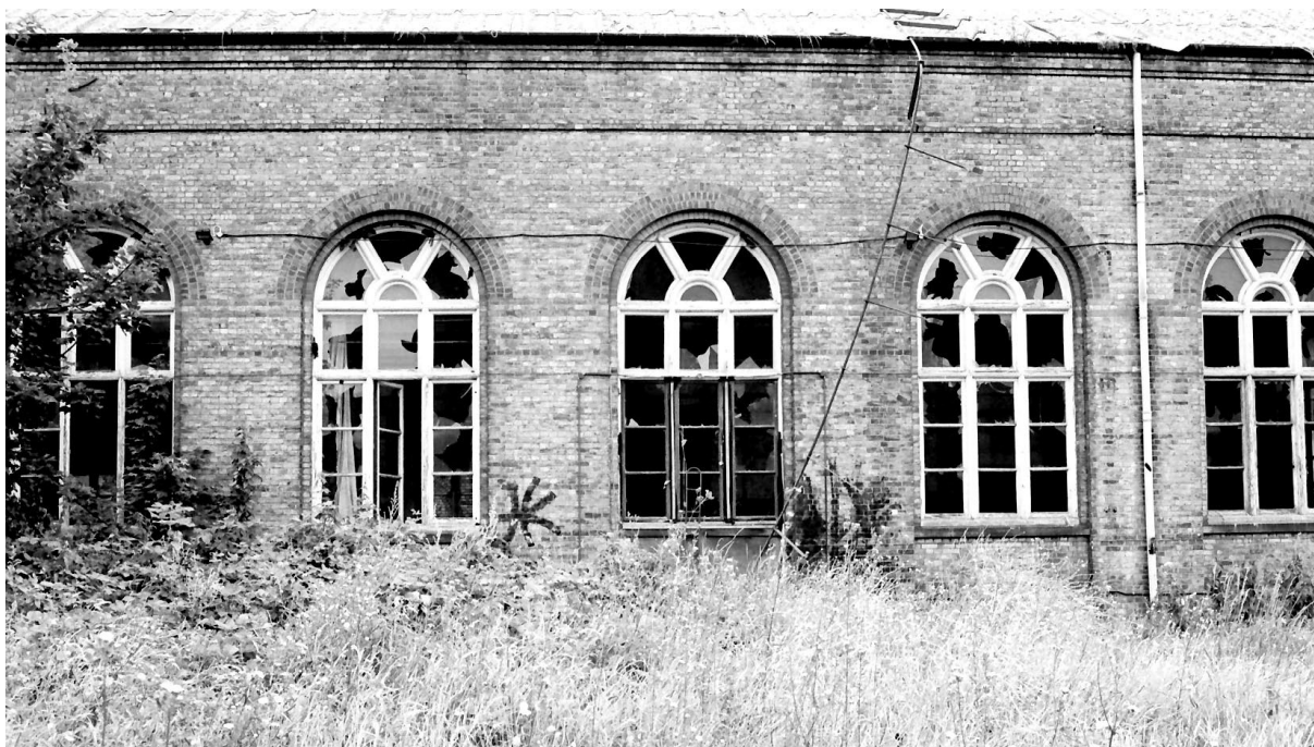
Figure 6. The engine house viewed from the south yard.
