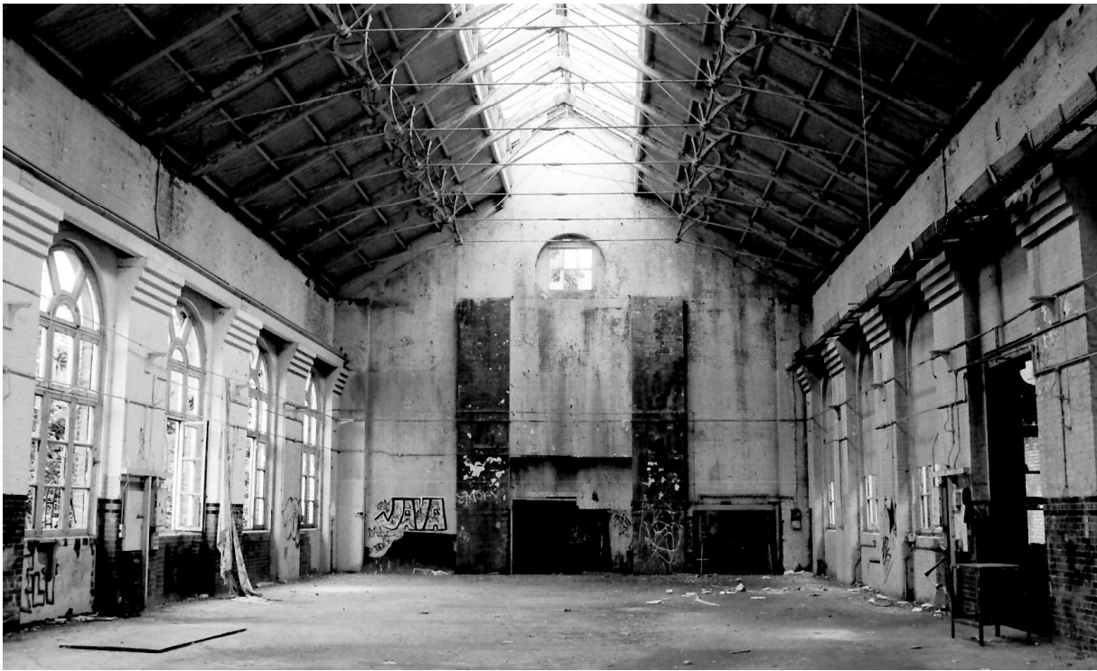
Figure 7. Inside the engine house looking towards the workshops. Note the tracks for the overhead travelling crane. The door on the right led to the boiler house.
