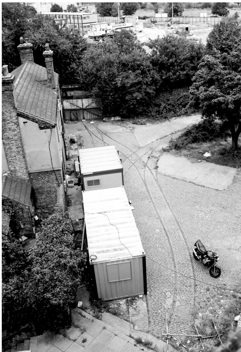
Figure 2. The yard to the south showing the foreman's house, left, and the 3-foot gauge tramway from Albion Dock, which entered the site through the gates at top left. The branch to the right led to the strategic coal store, which held 500 tons. Underneath the portacabin the tramway ran over a weighbridge.
