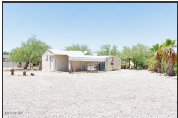
Utility shed/bunk house
