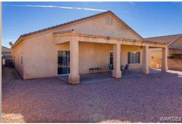
Back of property with a patio area and central AC
