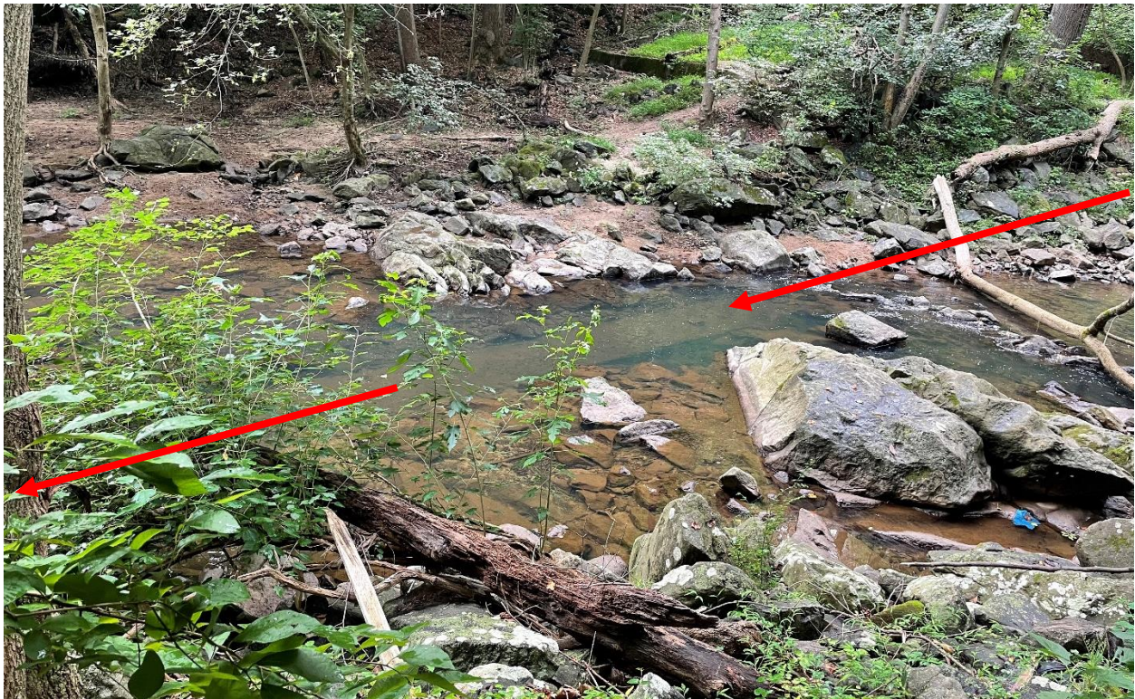
Sewer Pipe diagonal crossing one mile south of Burnt Mills
