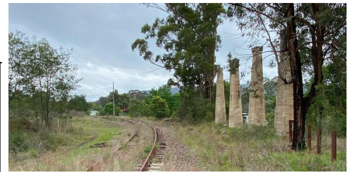
Figure 8 The four pillars at Bellbird - remnants of the old Bellbird Colliery - could be used as an historic feature with the future Bellbird Station.
