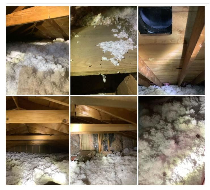
Attic Insulation: Insulation Type Fiberglass, Loose-fill
