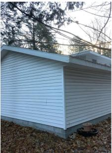
Siding, Flashing & Trim: Siding Material Vinyl, Brick Veneer
