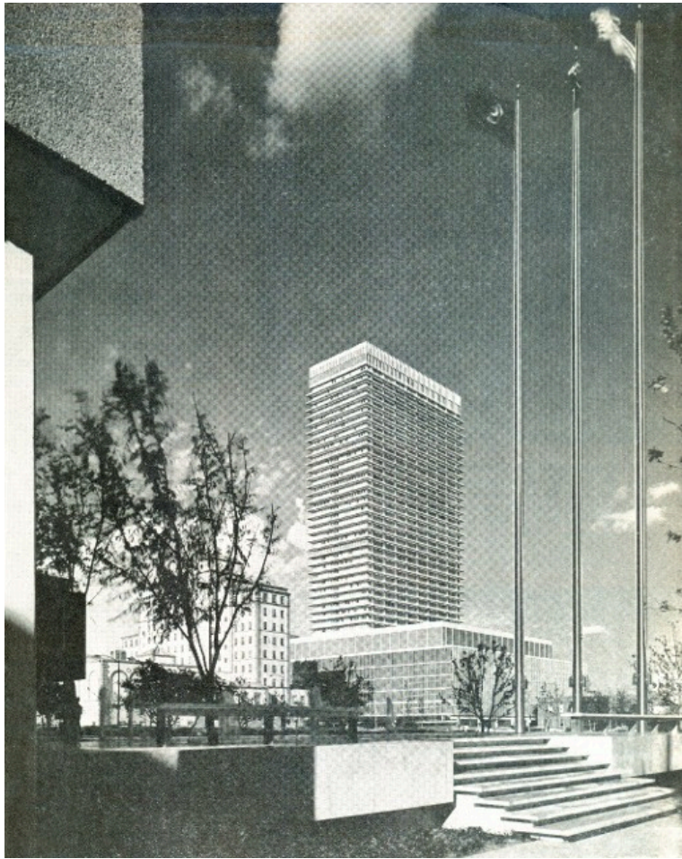
The HUMBLE OIL BUILDING was the home office for Humble Oil and Refining Company in Houston, Texas, was designed by Welton Becket with continuous horizontal sun shades on four exposures to reduce air-conditioning costs.
