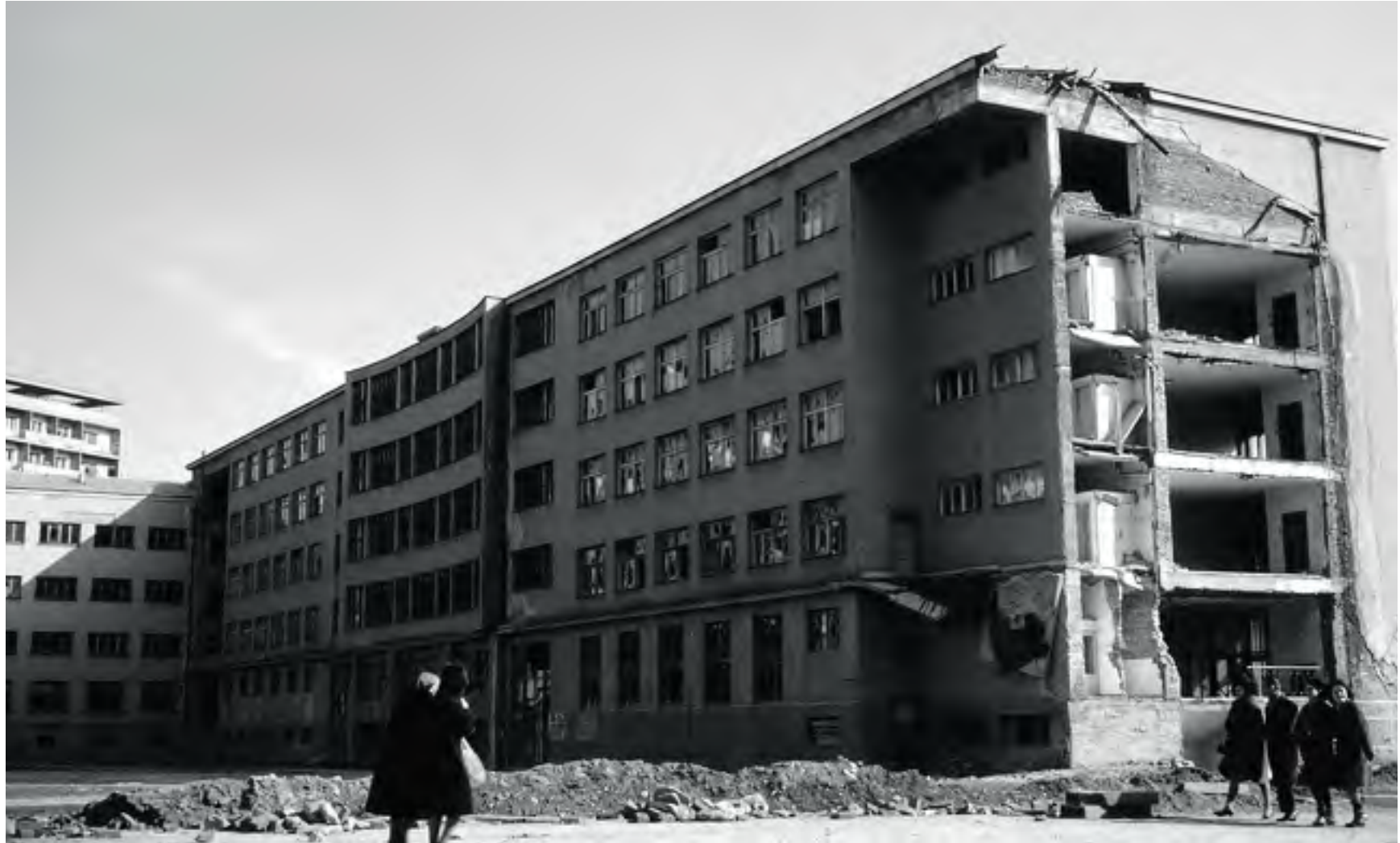
Aftermath of 1963 Earthquake Skopje, Yugoslavia, (Now Republic of Macedonia) Left 200,000 Homeless and Nearly 1,100 Dead
