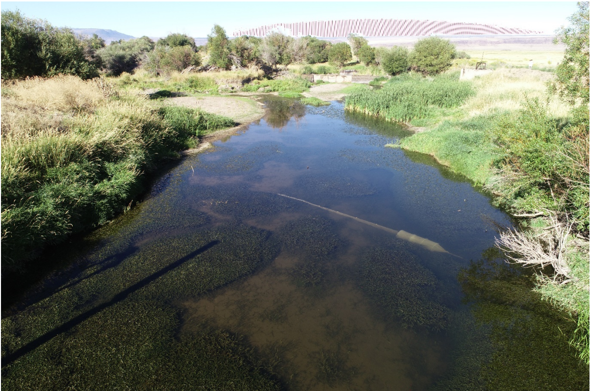
The forebay pool upstream of Starveout Diversion with hoop net set. photo credit Troy Brandt-RDG
