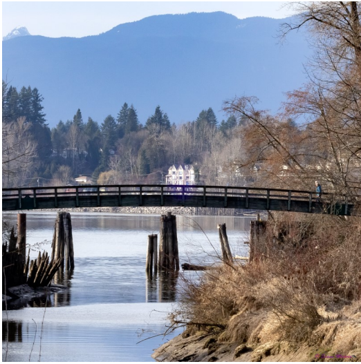
Bright River Bridge by Simon
