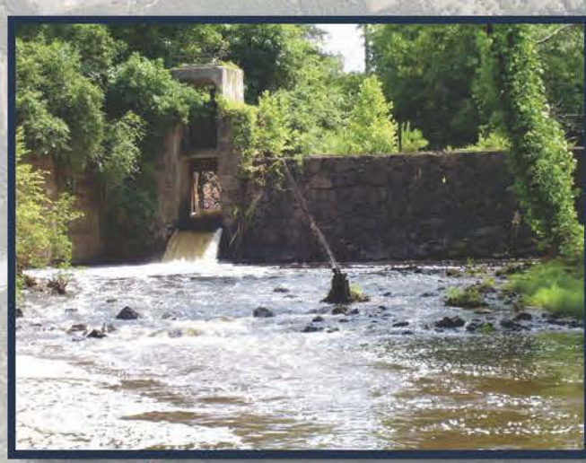
Steeles Mill Before Dam Removal
