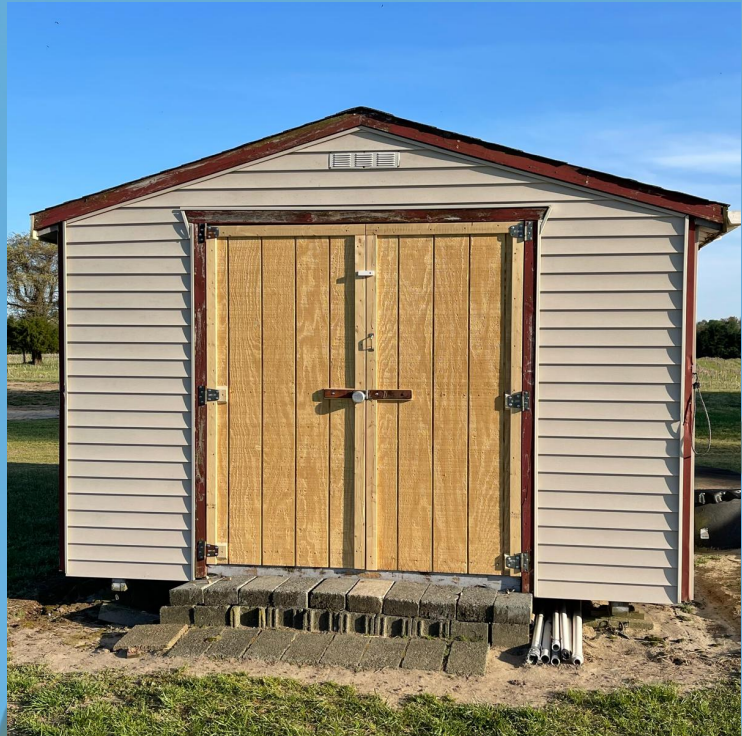
Nice job on repaired door. Thanks to Steve Rogers.
