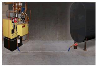
Surface view of a properly protected (sleeved) buried copper fuel line
