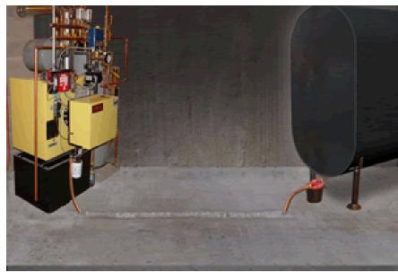
Surface view of an unprotected buried copper fuel line
