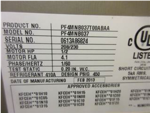
Air Handler Data Plate
