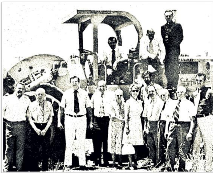
Demolition of the Church Building at 333 E. Virginia 1973
