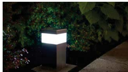
Bollard Pathway Bulb Replacement
