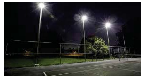
Area Lighting Bulb Replacement
