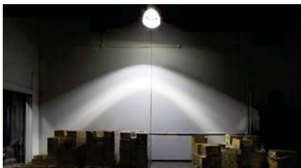
High Bay & Low Bay Bulb Replacement
