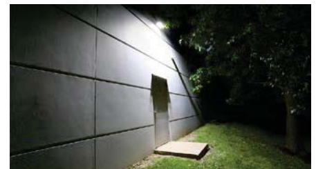
Wall Pack Bulb Replacement
