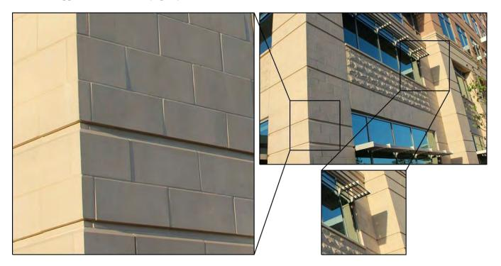
Notes: The photo on the left shows the large shadows that can arise from small, within specification, setting misalignment. The photo on the lower right shows the angle of the sun. Note that the stones on the side of the building in direct sunlight do not show any of these shadows.
