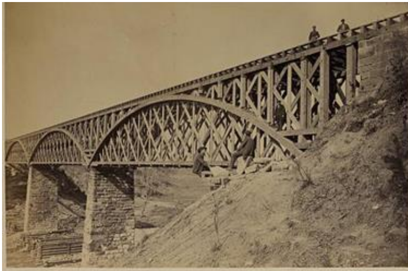
Rebuilt Bridge on Aquia Landing-Fredericksburg RR
