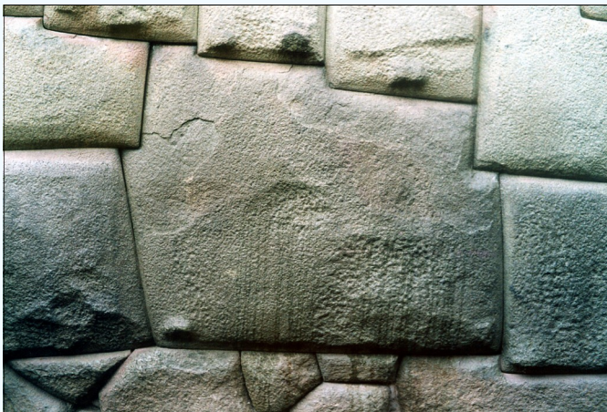
Incan masonry wall, carved of diorite bricks, in Cuzco, Peru Photo taken by Håkan Svensson (Xauxa) and used under Creative Commons License at Wikipedia https://commons.wikimedia.org/wiki/File:CuscoPiedra12angulo.jpg
