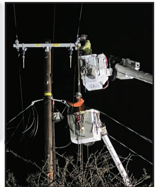
PG&E and arborists work in tandem late into the night to restore power on California St. after a large pine tree toppled over onto power lines.
