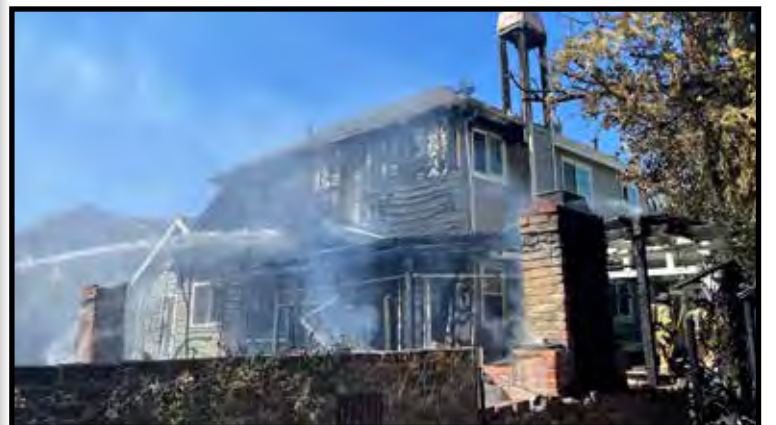
Just before noon on May 24th firefighters from Santa Clara County Fire Dept. responded to a structure fire on the 300 block of Harrison Ave. The fire caused significant damage to the detached structure at the rear of the property as well as causing damage to the house behind the property that was located on Central Ave. A small fire also started on a wood shake roof several doors away from the falling embers but was quickly extinguished. Photo: Courtesy SCCFD.
