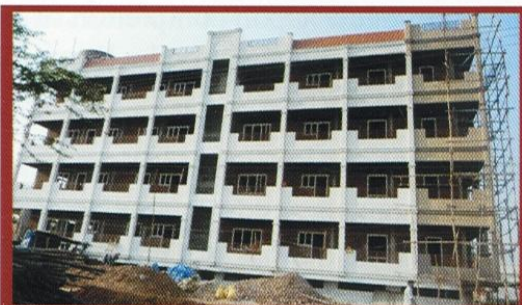
New school building in final stages of construction
