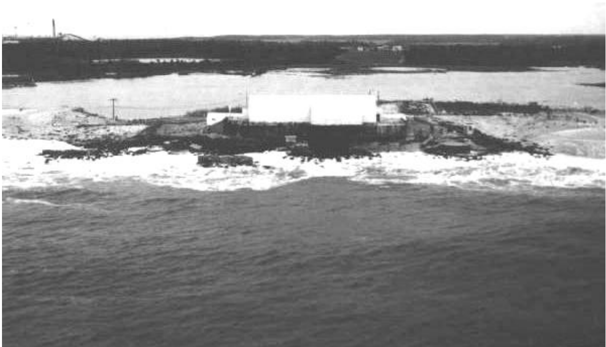
NAVFAC Cape May New Jersey (after the storm)
