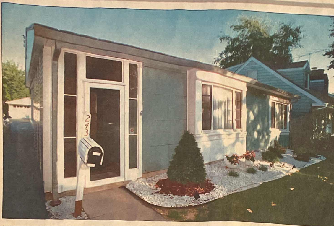
Lustron homes, such as this one in Lombard, can be recognized by their 2-by-2-foot enamel-over-steel panels on the outside of the house. Tribune photos by John Dzekan
