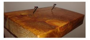
**Step 3:** Lastly, fully insert the shorter 2" screws into the predrilled angled holes on top of the shelf. **NOTE: Be Sure Not To Over Tighten When Inserting These Top Screws.** Over tightening could risk splitting the shelf. This will ensure that the front portion of the shelf will not slide off the rear piece. This completes your installation process. **LITTLE WOOD CREATIONS.**
