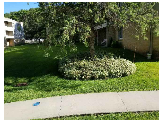
BLD #9 NE CORNER ROOF DRAIN
