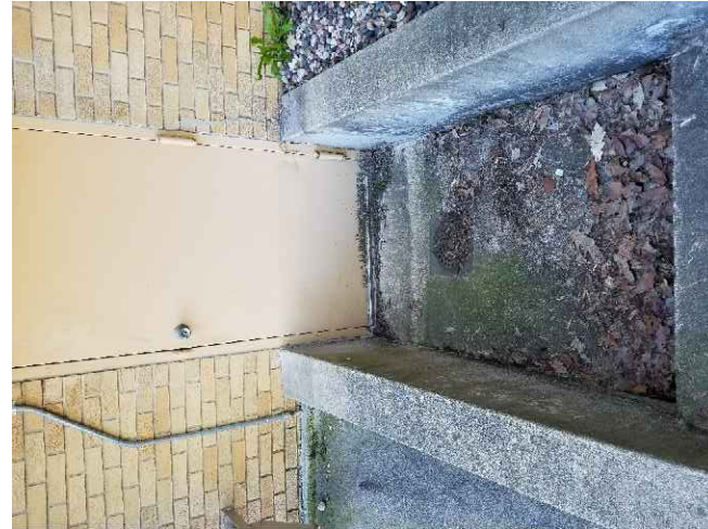
BLD #6 EAST INSIDE CORNER STAIRWELL
