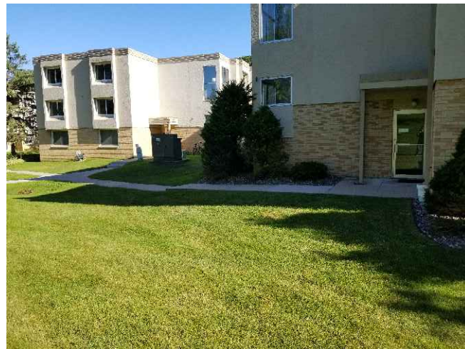
BLD #10 NE CORNER ROOF DRAIN
