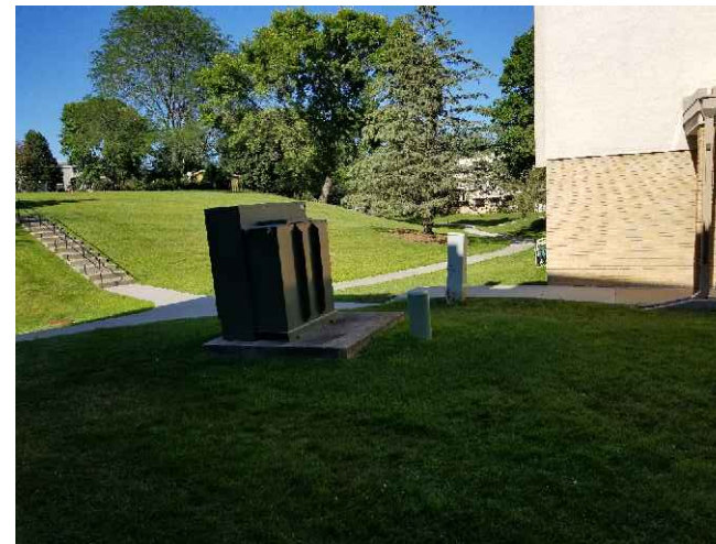
BLD #9 NW CORNER
