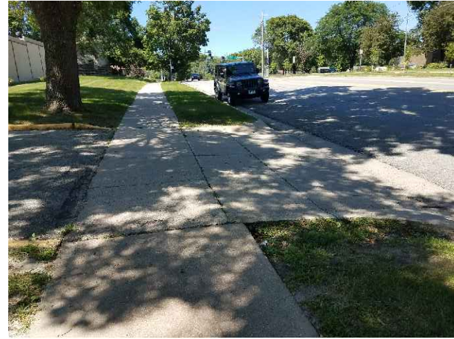
BLD #2 DRIVE APPROACH
