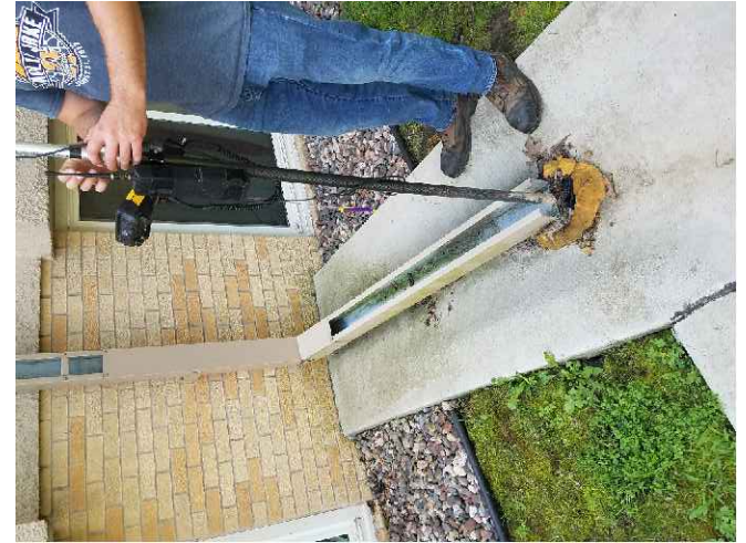
BLD #2 NORTH YARD INLET
