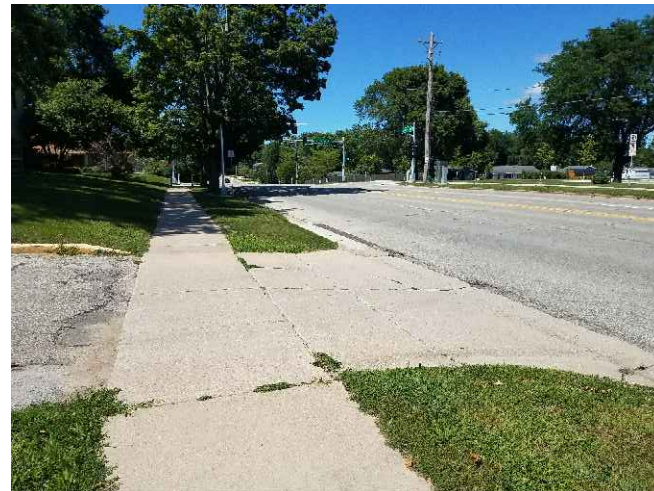
BLD #1 DRIVE APPROACH
