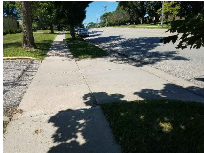
BLD #4 DRIVE APPROACH
