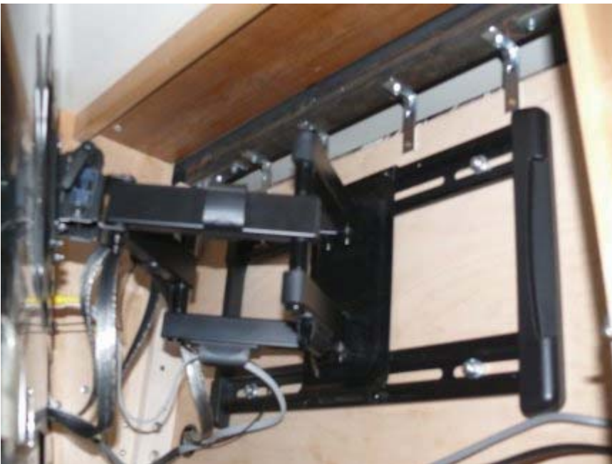
Flat panel TV pulled out from cabinet.
