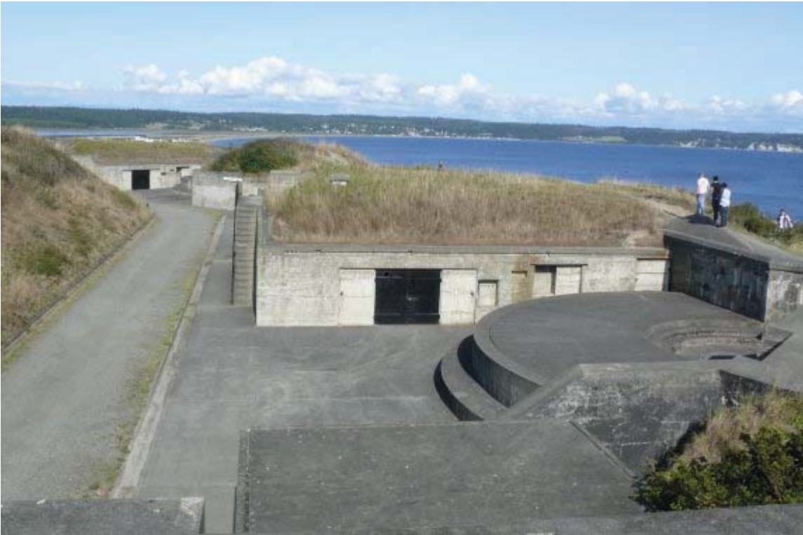
One of the abandoned 10 inch cannon stations.
