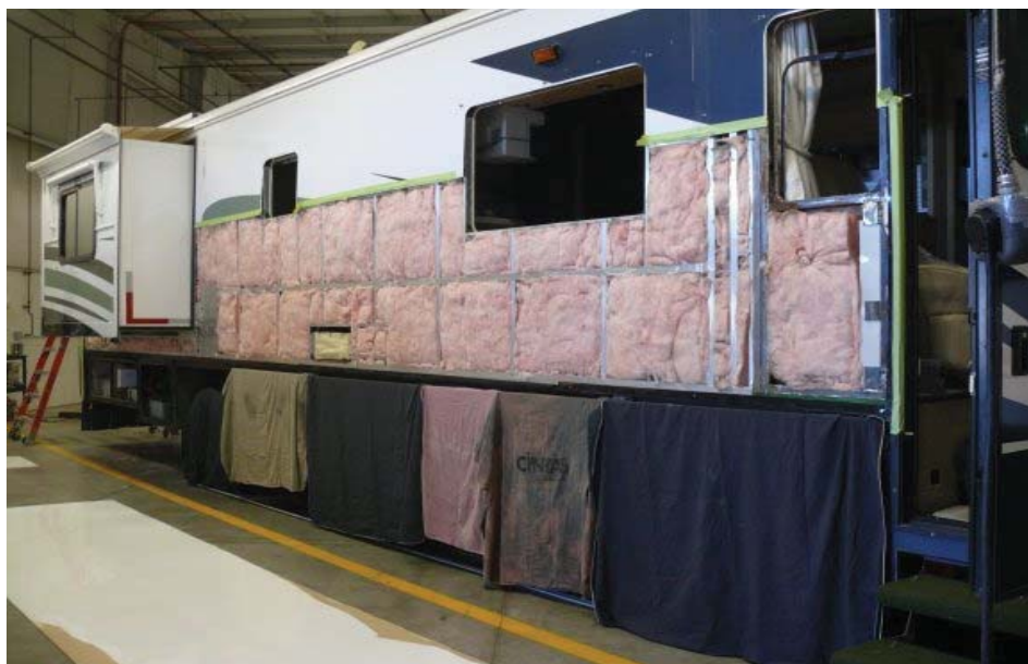
Our motorhome with a portion of outside wall removed.
