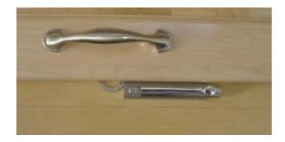
The above is an overhead cabinet in the every day unlatched position. To travel, we just slide the latch to the left and it covers the tab attached to the door. The same idea can be used horizontally or vertically.
