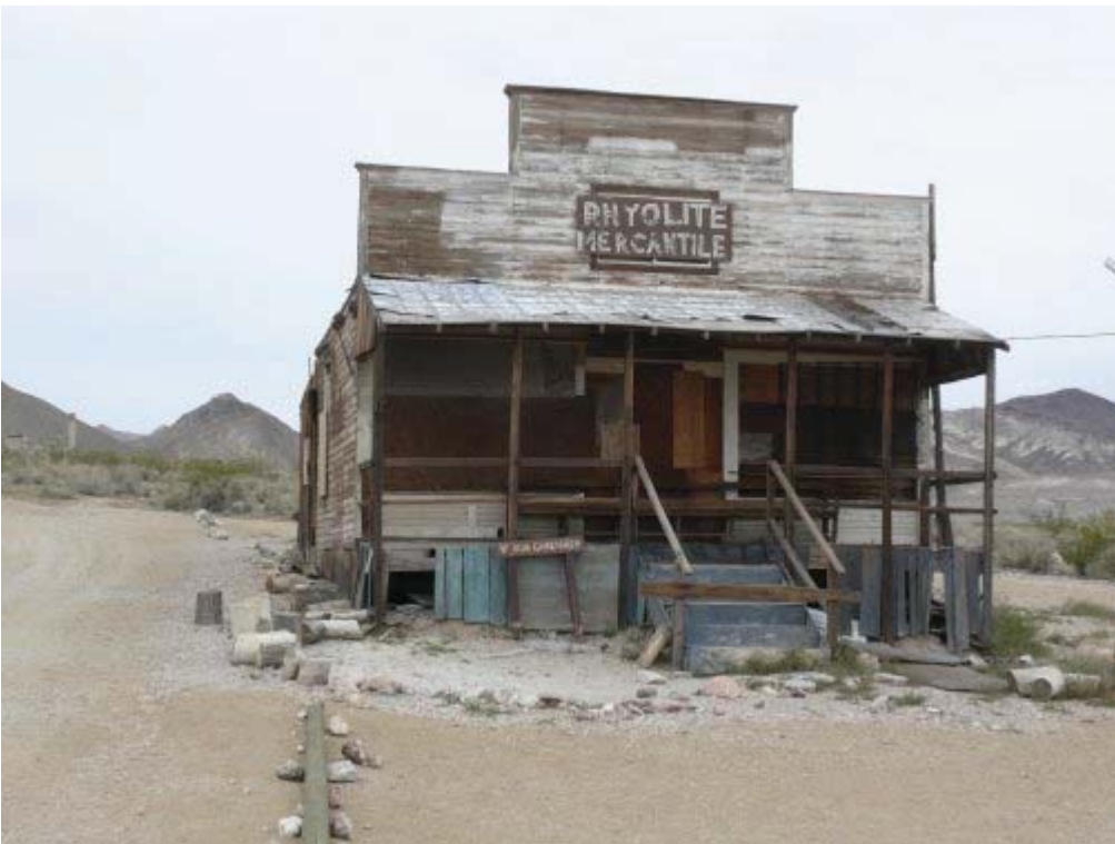
Rhyolite Mercantile building.
