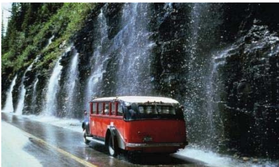
The "Weeping Wall" portion of Going-to-the-Sun Road.
