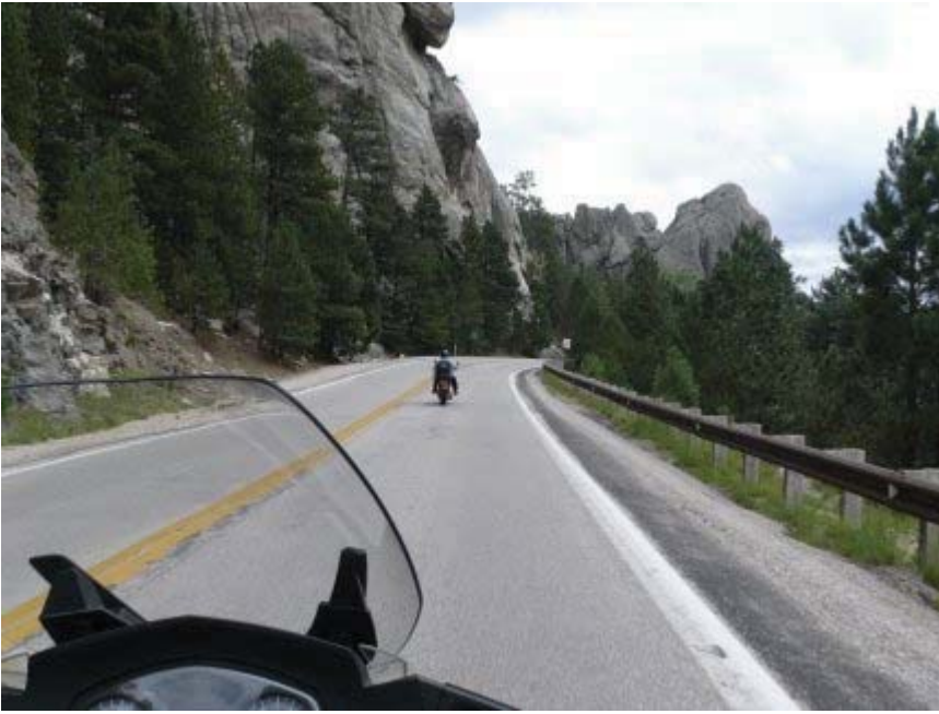
Iron Mountain Road.
