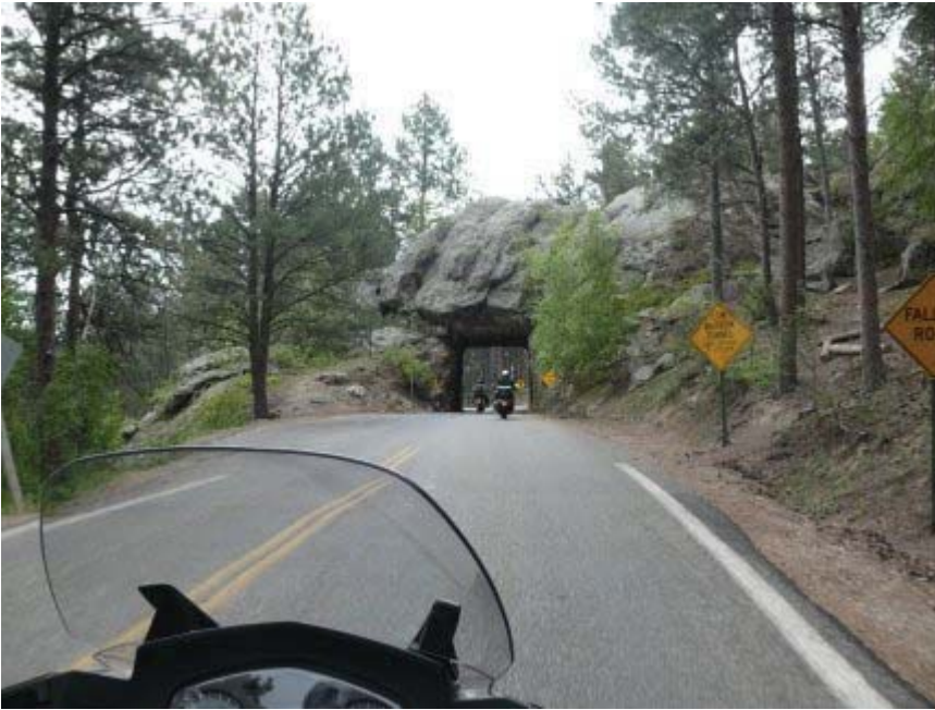
Two lane road with narrow tunnel.
