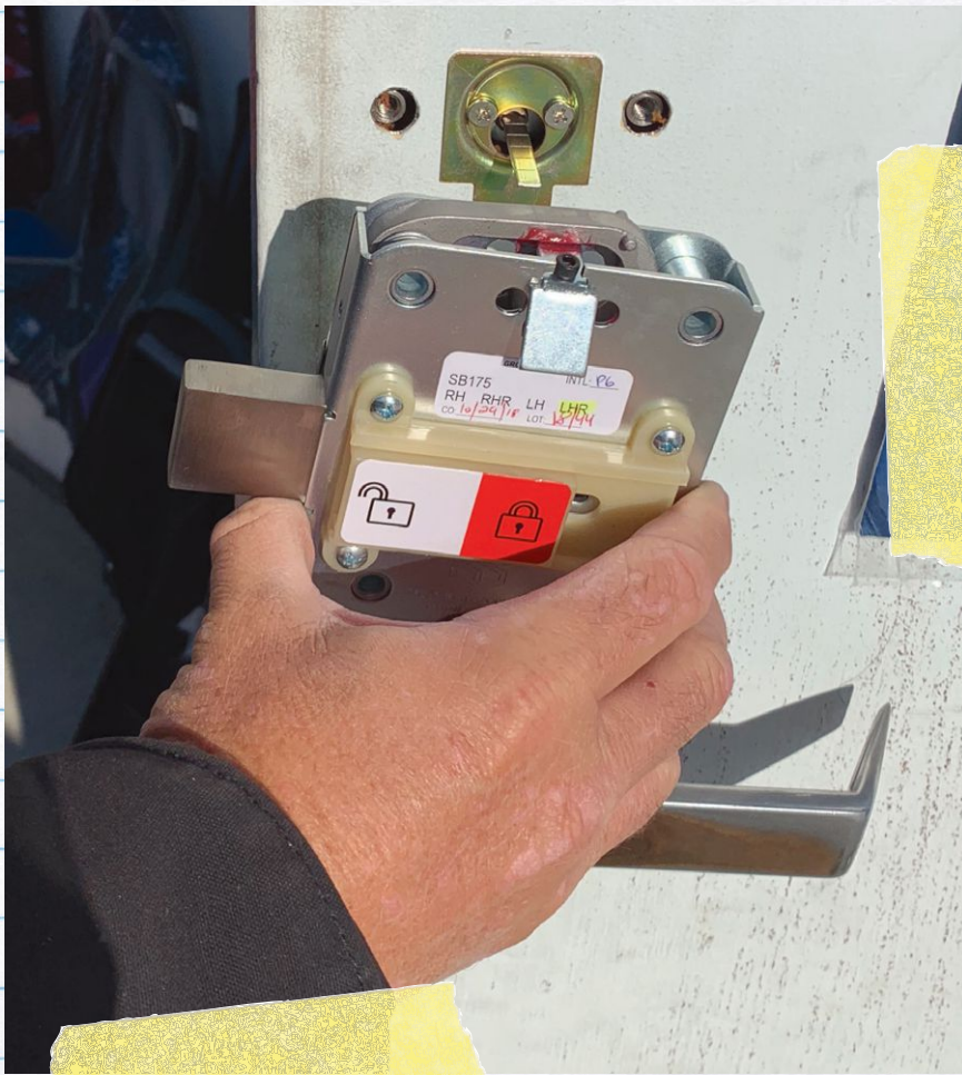
Installing a mechanical lockdown device.
