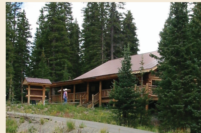
VISITOR CENTER VIEW FROM LOWER PARKING LOT PHOTO: GRAND MESA BYWAY ASSOCIATION
