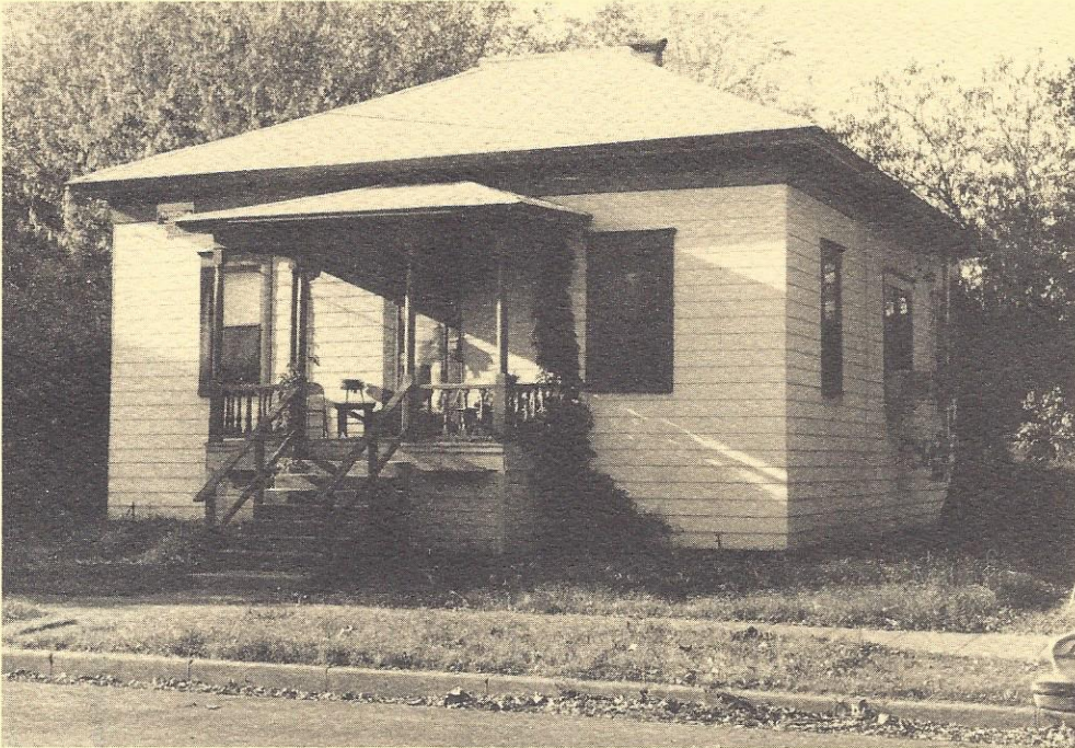
Soon To Be Rehabilitated
